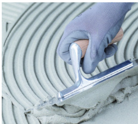
Spreading Adesilex P9 white
