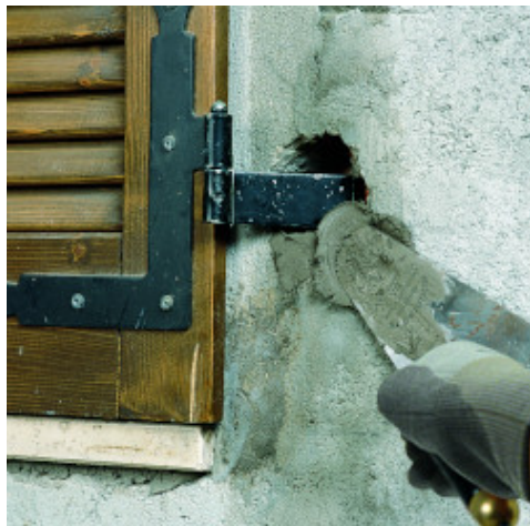
Fixing foundation bolts for windows using Lampocem
