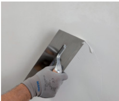
Part of application cycle for Mape-Antique FC Ultrafine
