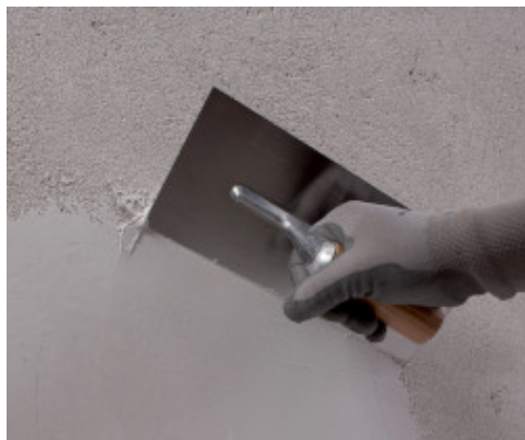
Spread on a first layer of Mape-Antique FC Ultrafine
