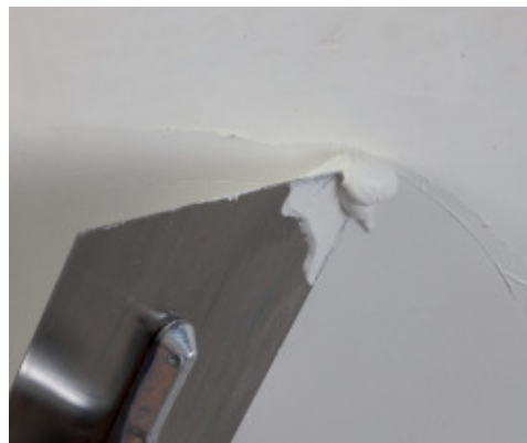
Smoothing over the product with a flat metal trowel
