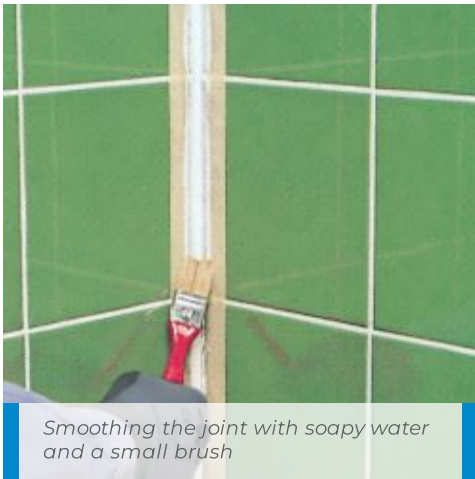
Sealing ceramic tile floor with Mapesil AC
