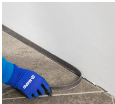
Once the grout has hardened, trim the perimeter of the Mapesonic Strip to remove the excess
