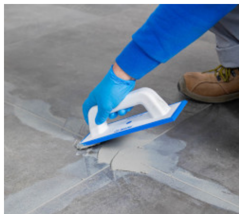
Grout the surface of the room
