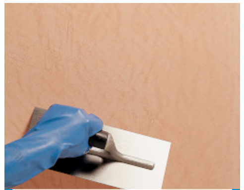
"Veneziano" effect: glossing of Silexcolor Marmorino with edge of a stainless steel float
