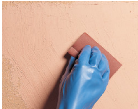
"Encausto" effect: sand-papering of Silexcolor Marmorino with a fine grained abrasive sand paper
