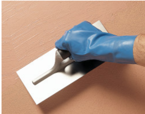
"Encausto" effect: application of Silexcolor Marmorino on Silexcolor Tonachino
