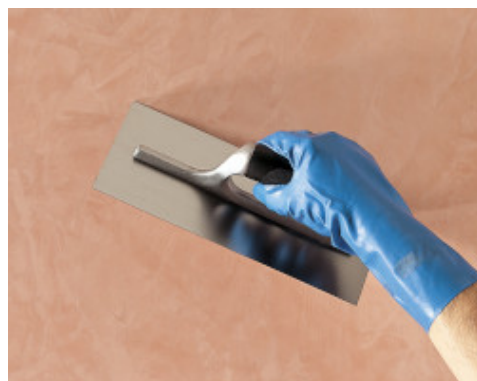
Classic effect: glossing of Silexcolor Marmorino with edge of a stainless steel float
