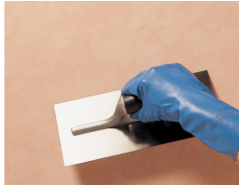
"Encausto" effect: glossing of Silexcolor Marmorino with edge of a stainless steel float
